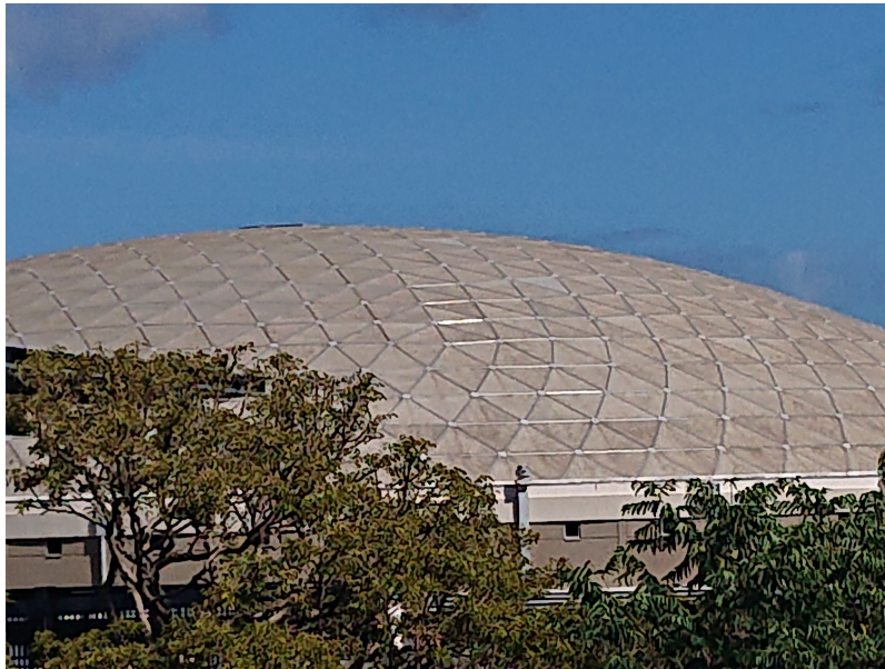
Figure 1.1: An example of a geodesic dome which should have Gaussian curvature approximately equal to the constant function 0.0004m^{-2} and mean curvature approximately equal to the constant function 0.02m^{-1} .
